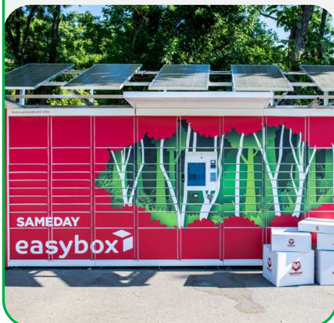
31 easybox lockers powered by solar energy
